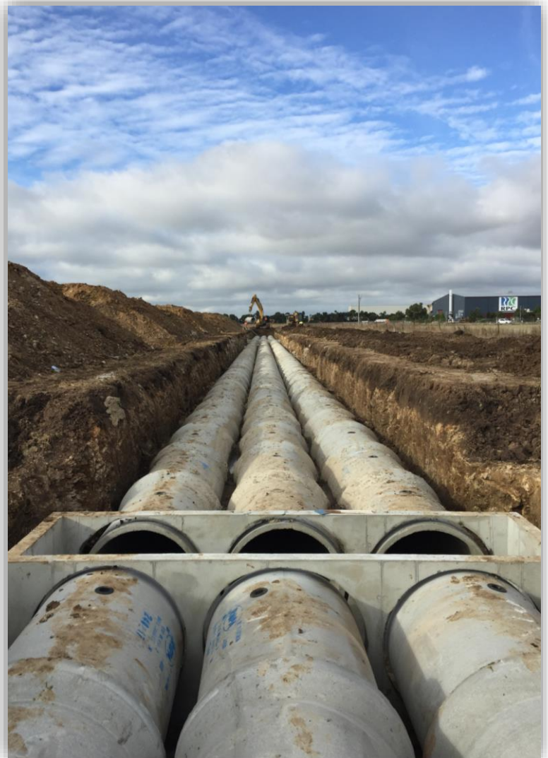
Triple 1500 RCP Pipe Installation
