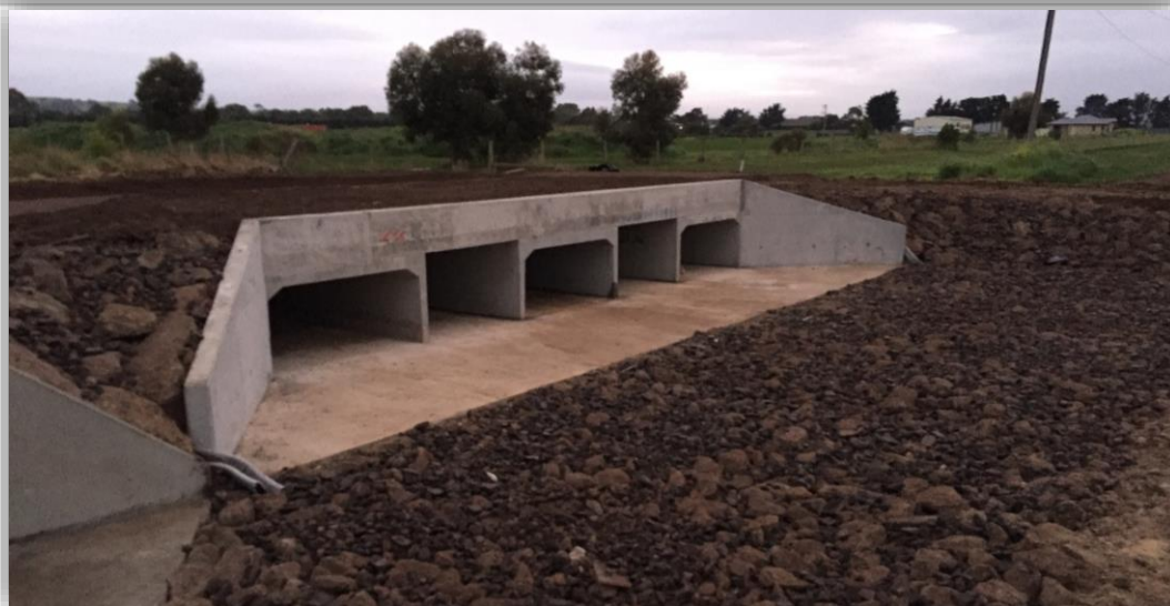
5 Cell Culvert Structure
