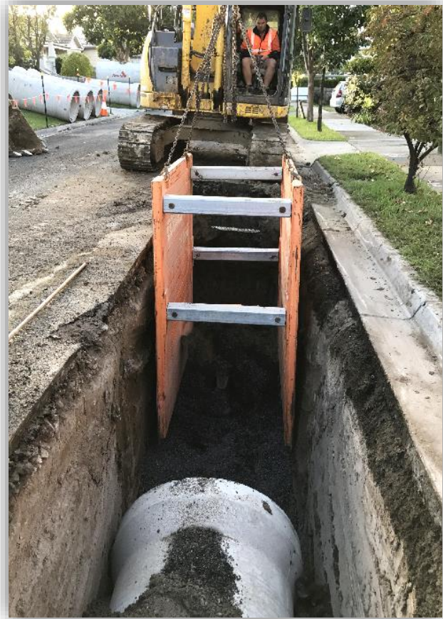
Construction of DN900 RCP Drainage
