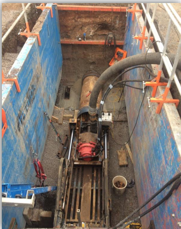
DN525 Trenchless bore between residential properties
